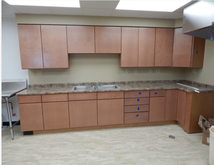
New kitchen cabinets
