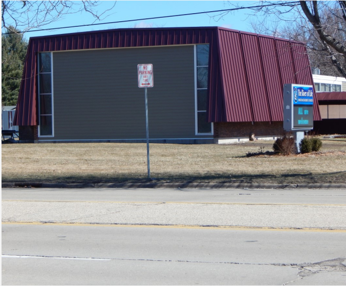
Sanctuary with new siding
